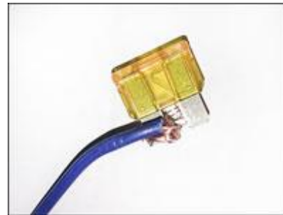
Wire Jammed Into a Fuse
