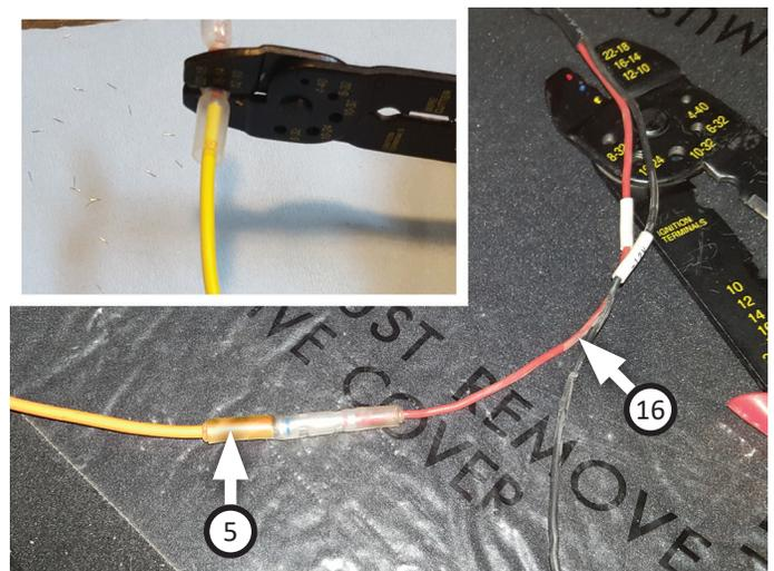
14. Place **female quick disconnect (15)** to remaining end of controller kit. Crimp connector to secure wires together.
